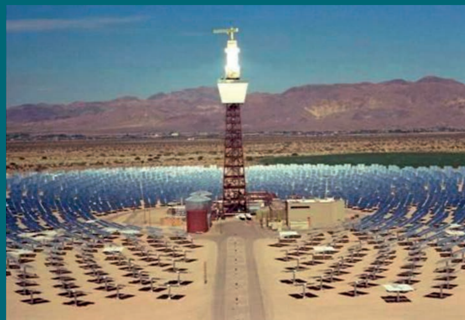
Figure 2.3.7 An example of solar power plant with central tower
